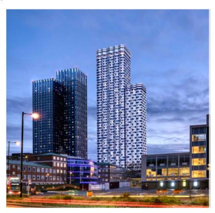
3.2 The applicant proposes to construct the scheme as a modular building, meaning that each 'module' will be manufactured off site in a controlled manufacturing environment. The modular build method offers a wide array of unit types and incorporates a bespoke, contextual and crafted façade design. It would also allow the applicant to construct the
